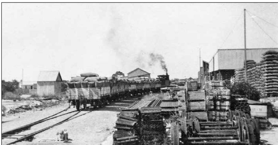
*Left: The way it was: this photo from the Eric O'Connor Collection shows bagged grain in small open C wagons in Port Lincoln yard, in the 1923-26 period. Note also the large bagged grain stacks on the right.*
