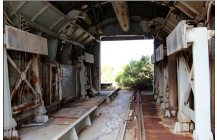
Above: inside the tippler building, 21 March 2014.
