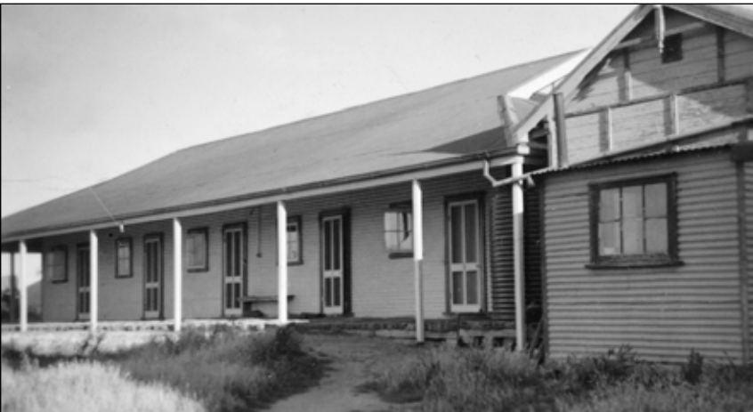
This photo shows the 1927–1969 barracks at Thevenard. The Simplex building with its distinctive outside framing can be seen in the top right of the image, behind the small corrugated iron structure in the foreground.
